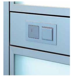
Specially developed lights with an adapter for the system grooves were integrated into the walls at several places. The power supply is concealed in the system wall. Operating switches are also part of the system.
